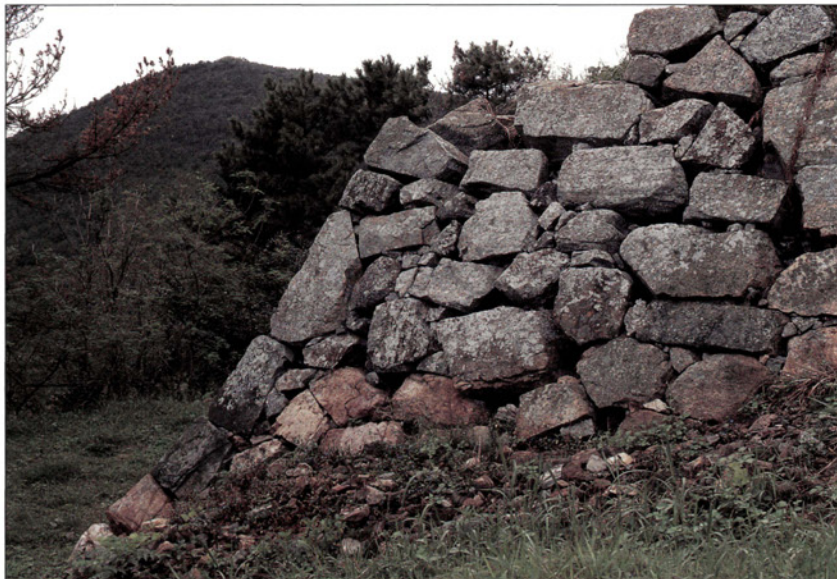
The sloping stone wall of the keep of Gijang, typical of the native Japanese design imported into Korea as the wajo .
