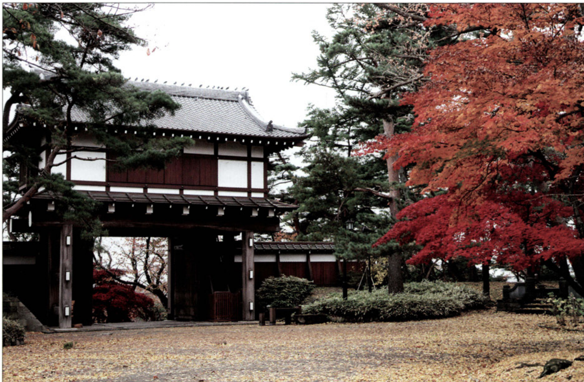
A comparatively simple gatehouse is shown here at Kubota Castle in Akita in northern Japan.
