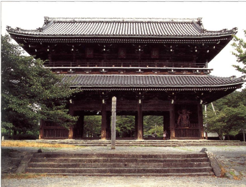
The Nishi Daimon (western great gate) at Negorodera is a gateway with no walls or gates, as befitted the peaceful times when it replaced its predecessor. The previous gateway would have been easier to fortify.
