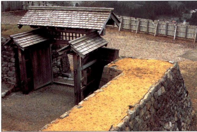
The gateway and koguchi (barbican) that defend the perimeter of the hon maru at Torigoe.
