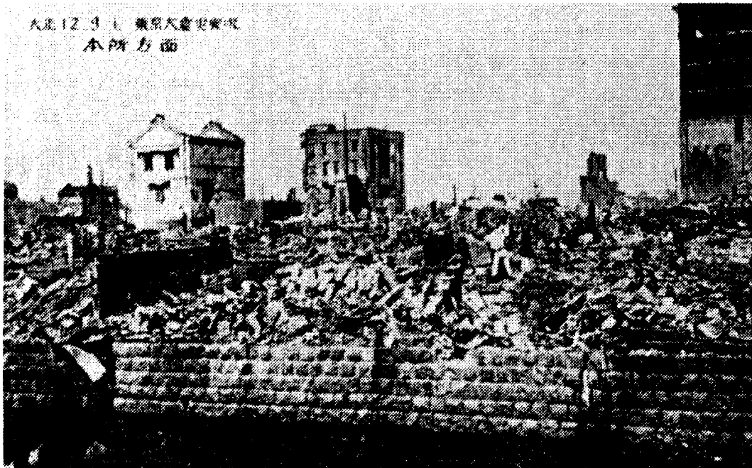
13. Honjo ward in the aftermath of the 1923 earthquake.
