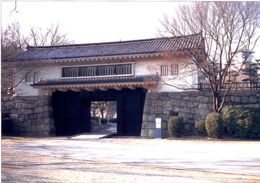
A two-storey gatehouse of Osaka Castle with a very solid set of gates.
