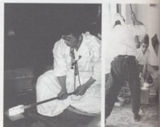
When heated to high temperatures, the lump of steel glows yellow, at which point it is hammered and forged into a small block by the swordsmith and his assistants.
