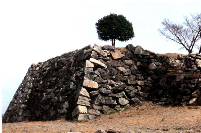
The base of the keep at Sunch 'on. Like most of the Wajō sites, Sunch 'on was built in traditional Japanese style by excavating the natural hill to give a series of overlapping baileys reinforced with stone. A rudimentary keep would have stood upon this carefully shaped stone mound.
