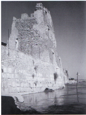
All that remains of the 12th-century Saljuq palace in Mosul is a reception hall or throne room overlooking the river Tigris. (Author's photograph)
