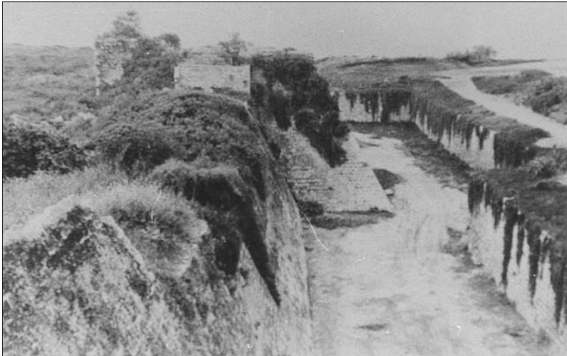
The excavated outer defences of Caesarea Maritima on the Palestinian coast clearly show how the moat of the refortified city followed the line of the wall precisely. The sloping lower part of the city wall is on the left while the near-vertical retaining wall of the moat is on the right.
