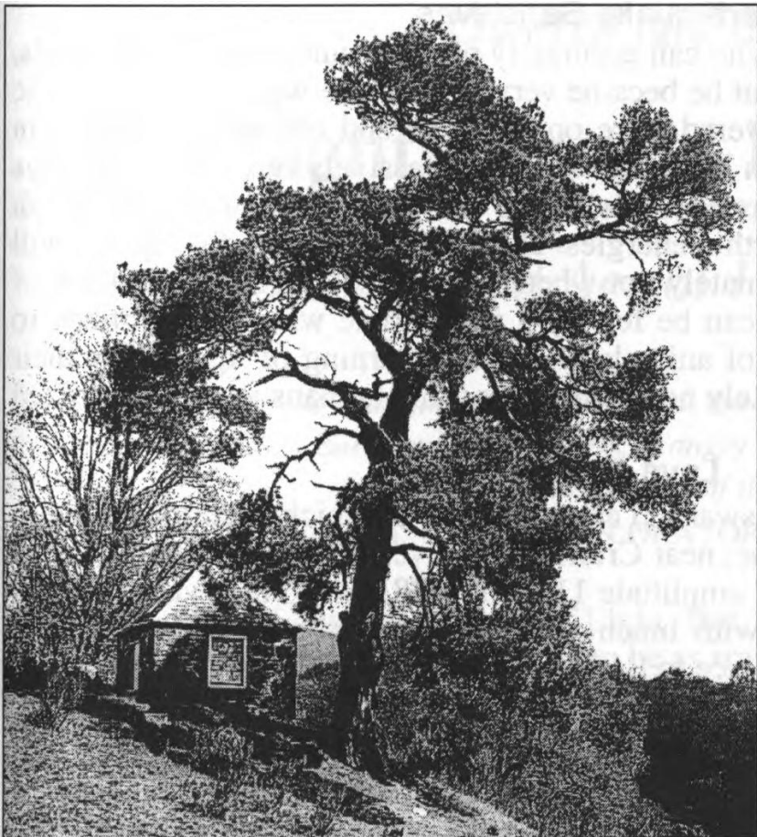
Fig. 76. The "Earthquake House" in Comrie, Scotland. This is where the world's first seismometers were installed.
