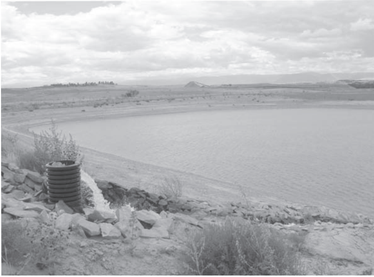
Pond disposal (a)
