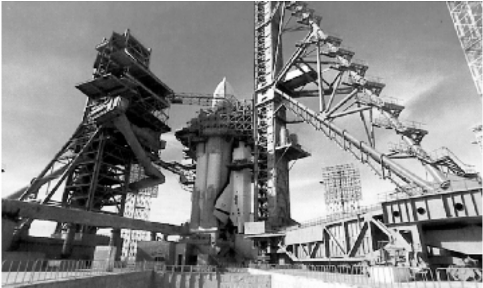
Pad 37 with the 145 m high rotating service structure in place ( source: www.buran.ru ).
