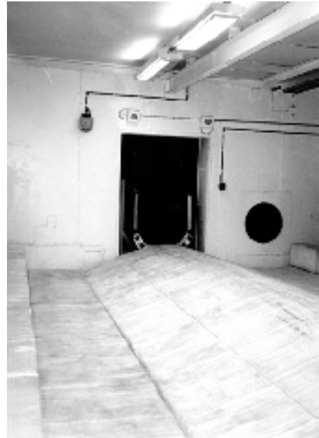
Underground room where the emergency chute ends ( source : Edwin Neal Cameron).
