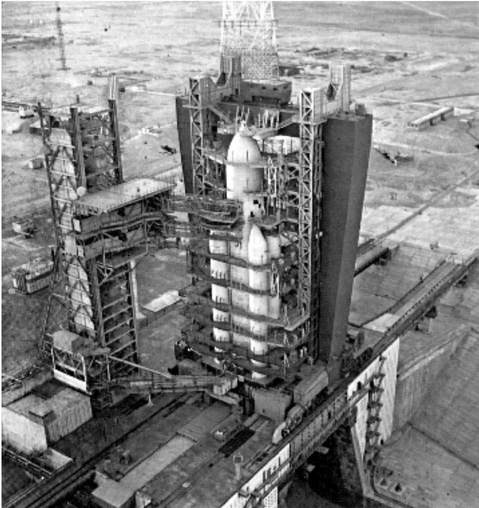
Energiya test model on the UKSS ( source: Mashinostroyeniye ).
