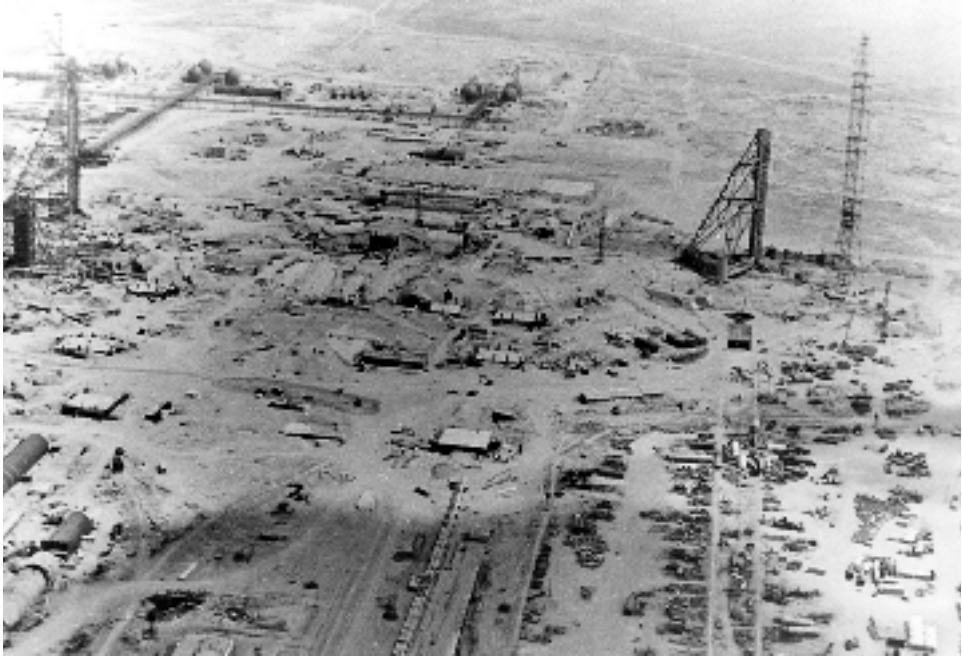
N-1 pads being rebuilt for Energiya-Buran (B. Hendrickx files).
