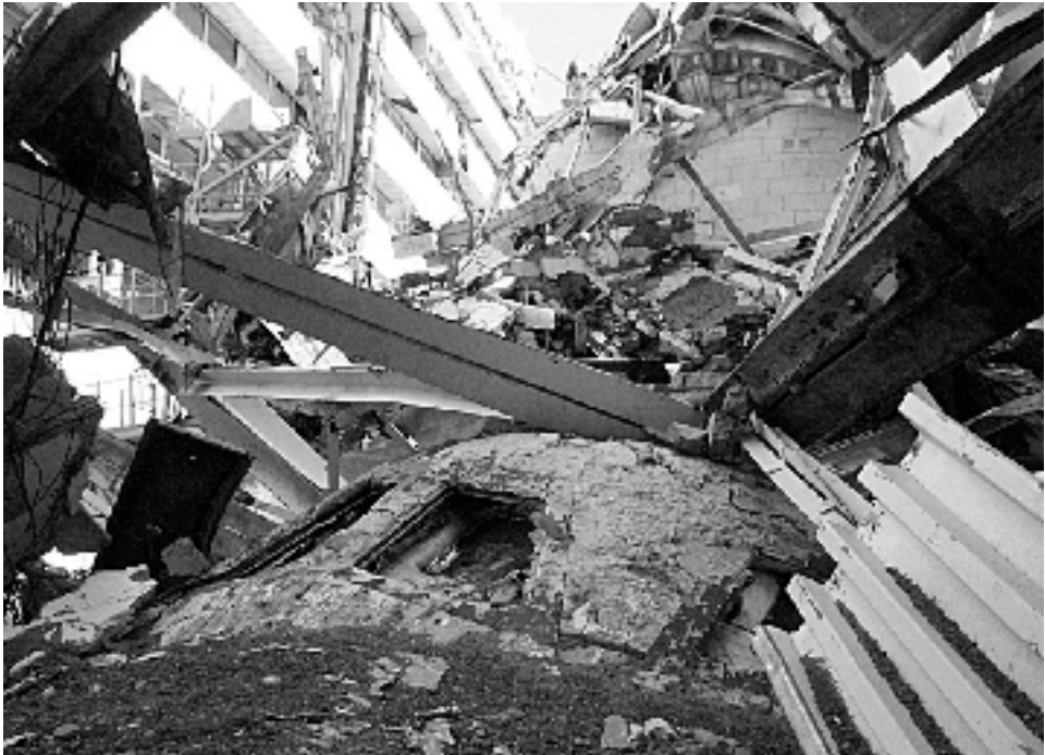
Remains of Buran after the roof collapse ( source: www.buran.ru ).
