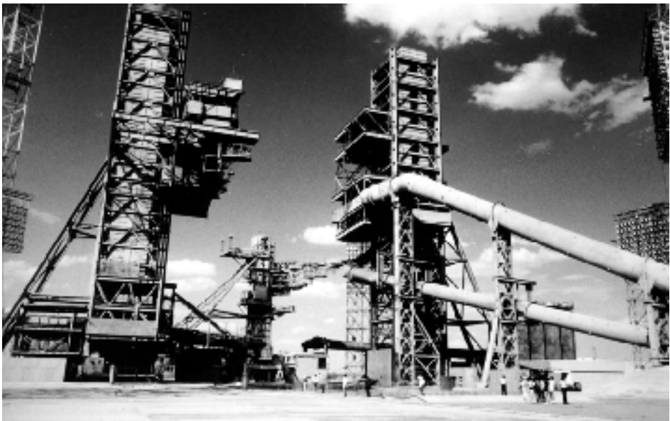
Pad 37 with shortened rotating service structure (B. Vis).
