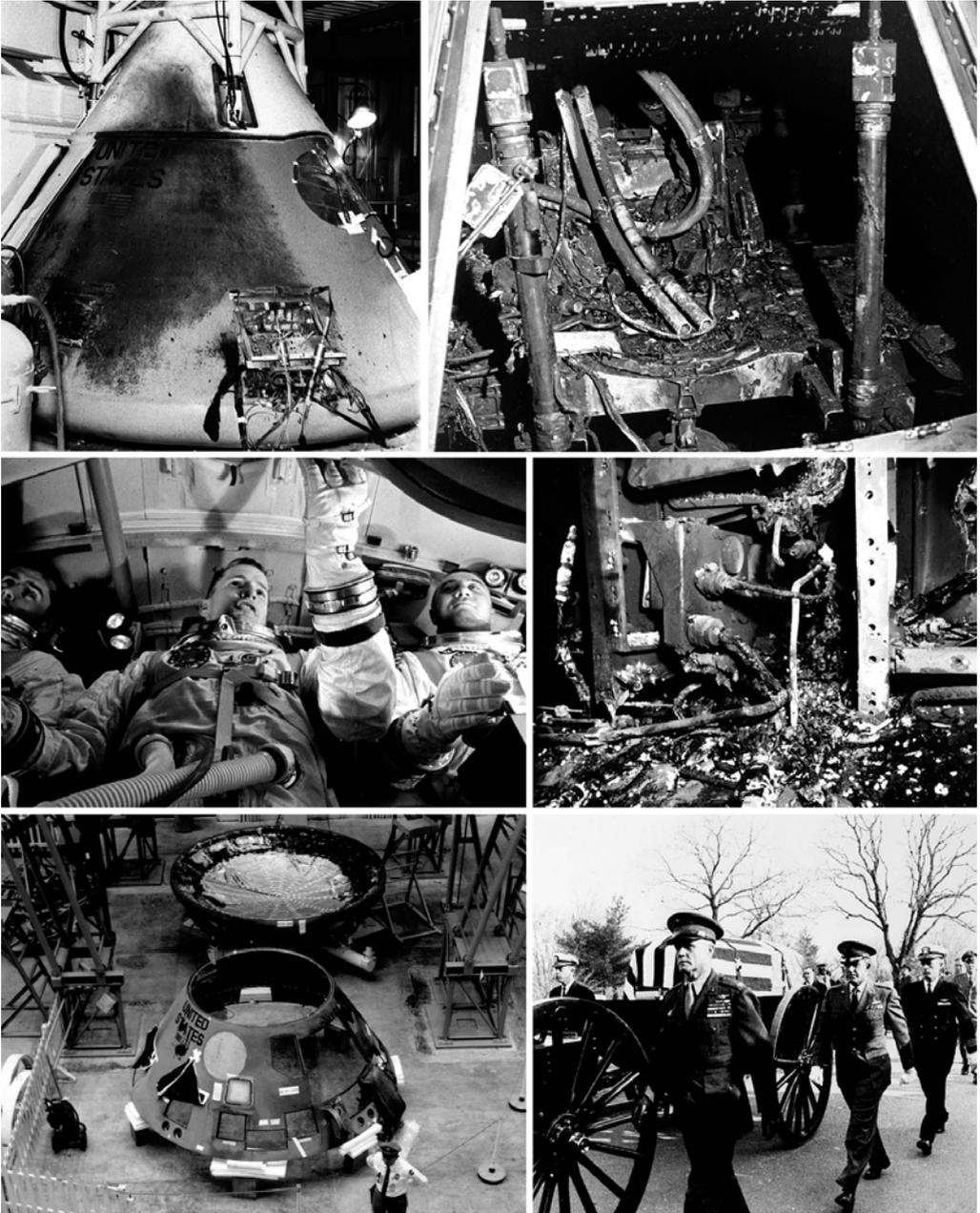
The exterior of the fire-damaged Apollo 1 command module in which Grissom, White and Chaffee died (top left); a view through the hatch; the crew positions, with the hatch above the center couch; the vicinity of the environmental control unit, where the ignition source is believed to have been; and its disassembled outer structures. John Glenn, Gordon Cooper and John Young escort Grissom's coffin.
