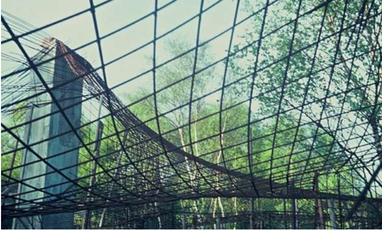
Figure 2: Steel lattice attached to the chimney.
