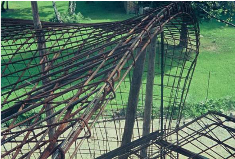
Figure 3: Steel ‘girders’ at the edge.
