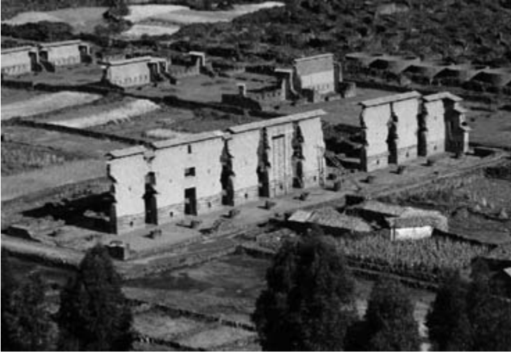
Figure 5.1 Photograph of the surviving central wall of the large Inka building, the ‘Temple of Viracocha’, at Raqchi. The small tile roof is a modern conservation measure, but the stone base, the 12 m high mud brick wall and the footings for the columns are original. (Photograph by Bill Sillar.)
