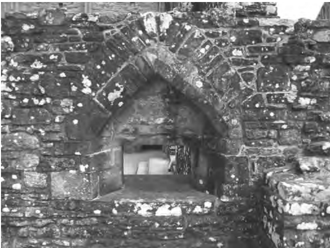
4. Serving hatch. Tintern Abbey kitchens, Monmouthshire
