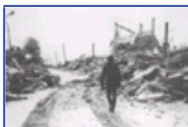
Figure 67-6 Main street in devastated Armenian village showing complete collapse of all buildings after Dec. 7, 1988, earthquake. (Courtesy Eric K. Noji.)
