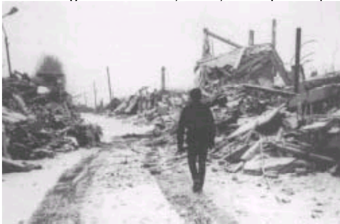
Figure 67-6 Main street in devastated Armenian village showing complete collapse of all buildings after Dec. 7, 1988, earthquake. (Courtesy Eric K. Noji. )
