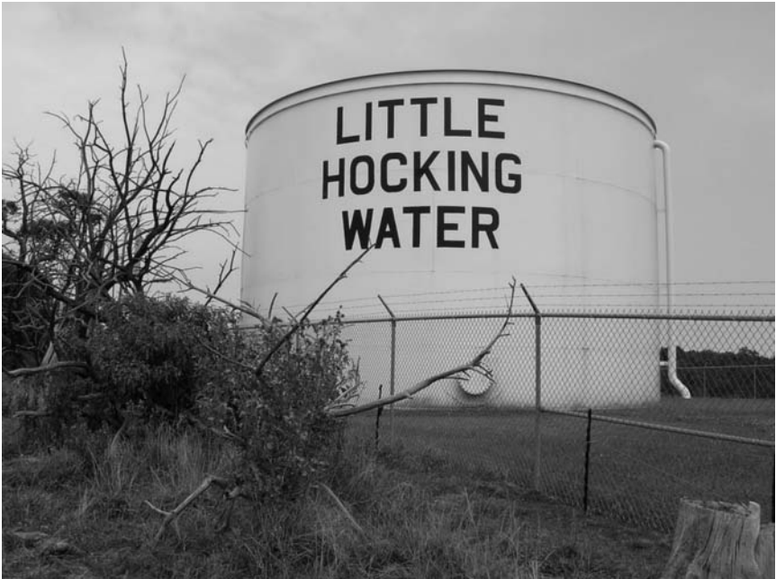
One of eight water tanks belonging to the Little Hocking Water Association.
