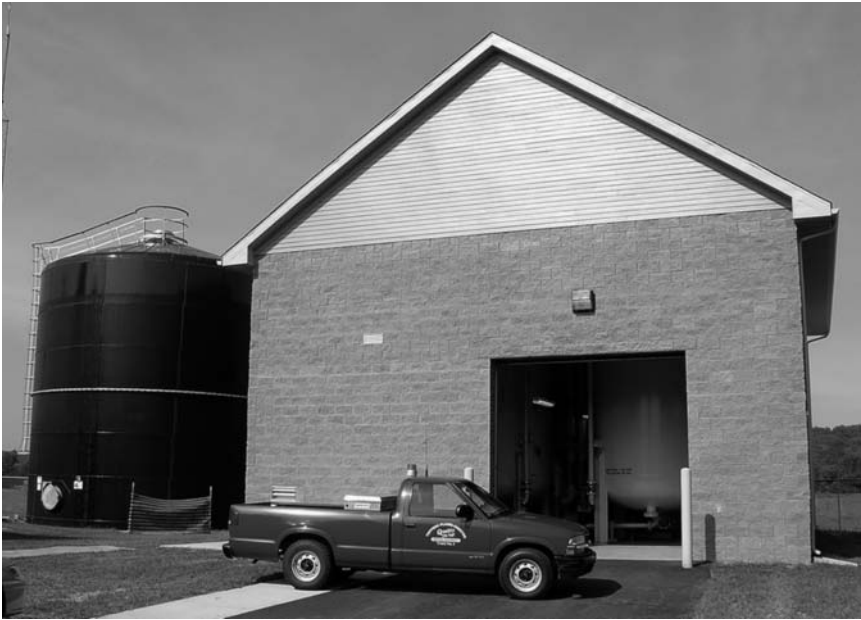
The blockhouse contains the GAC treatment system built by DuPont to filter out C8 for Tupper Plains.
