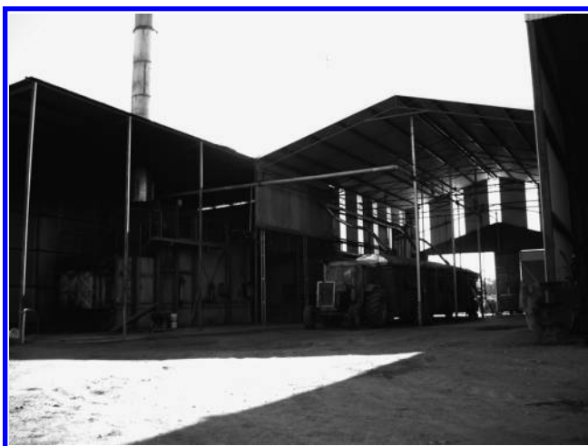
FIGURE 5.22 Distillation plant with container technique.
