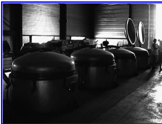
FIGURE 5.11 Battery of four distillation units.
