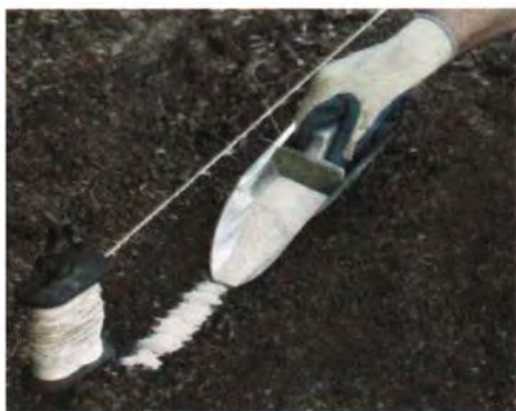
Measure out new garden beds with a string line or rope, then mark them with lime or sand.
