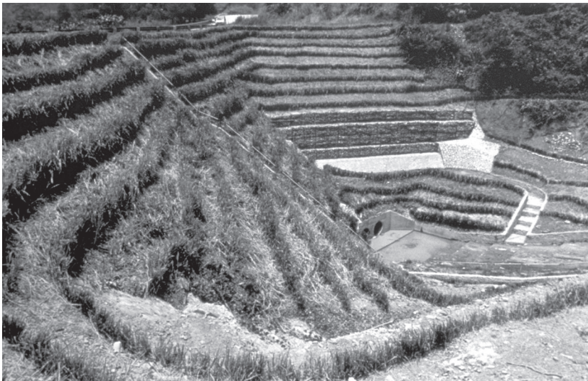
Figure 3.6 Terrace borders with vetiver grass.
