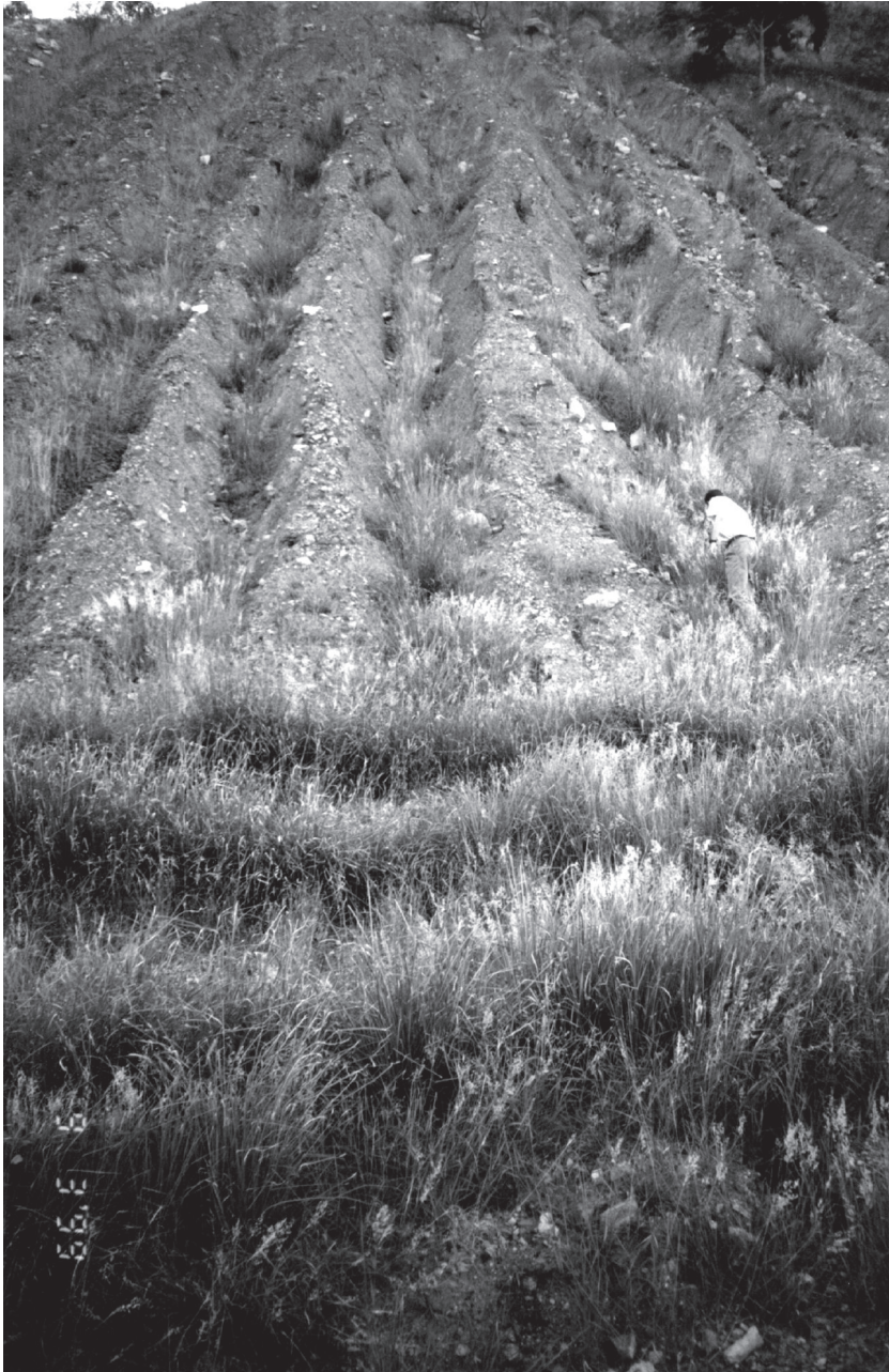
Figure 6.4 Vetiver is used to stabilise the deeply cut gullies of the overburden stockpile of an old coal mine (background) in Queensland, Australia. The horizontal rows in the foreground were planted to trap eroded material from moving offsite.
