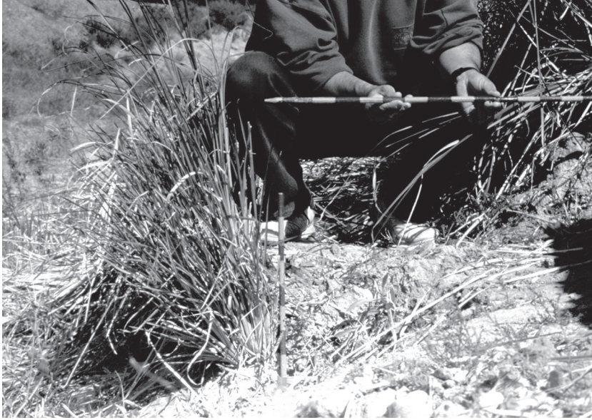
Figure 3.9 The distance of 1 vertical metre between the rows (height) is recommended in literature and has produced outstanding results in erosion control in the project carried out in Murcia.
