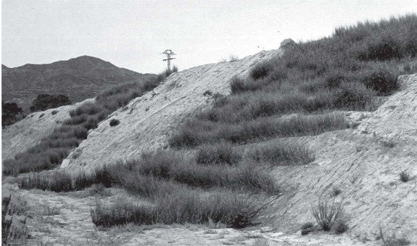
Figure 3.5 Vetiver plants are employed against erosion in embankments with a gradient of around 60%.
