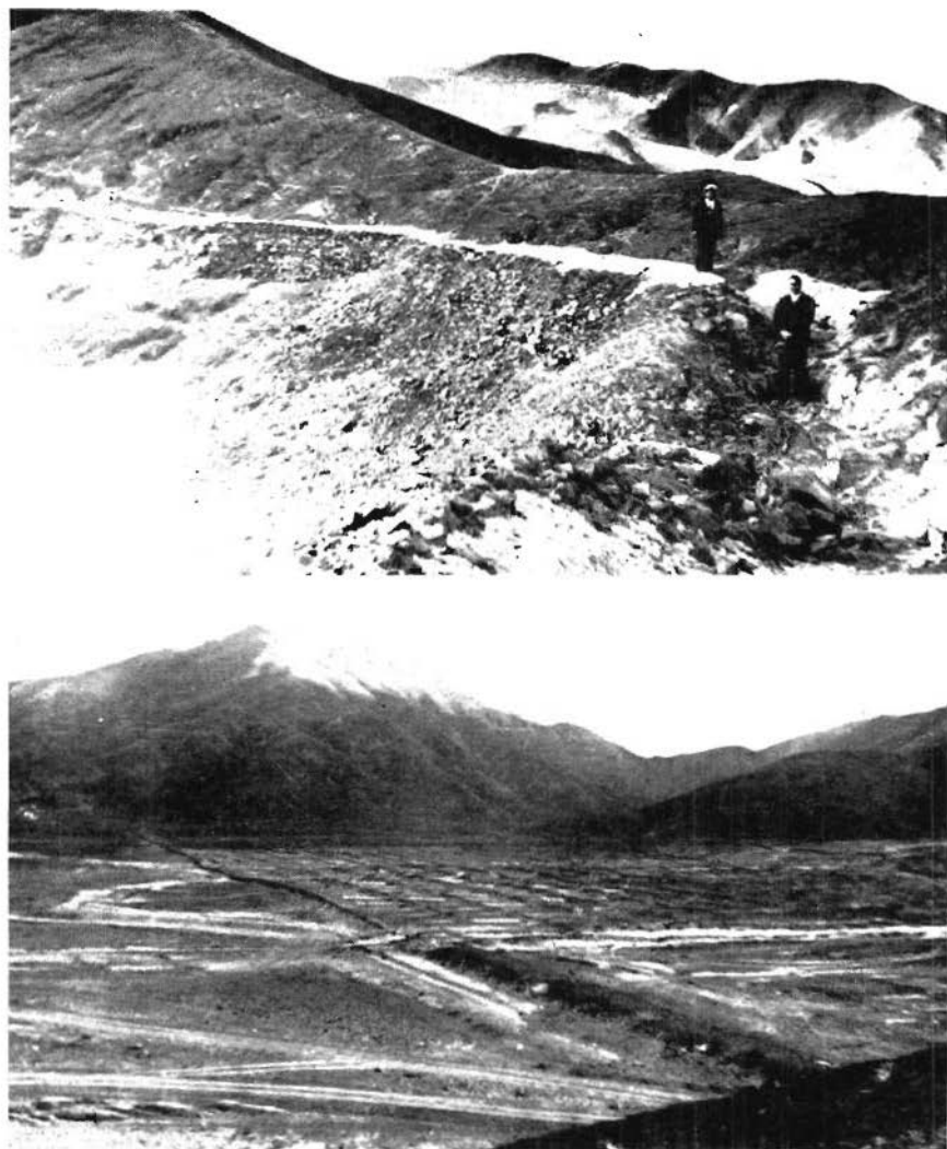
FIG. 79. The ancient civilizations of Peru had skilled engineers. In the upper view is seen one of the ancient aqueducts still intact for thirty-five miles which modern scientists estimate was capable of delivering sixty million cubic feet of water per day. They had no hardened tools or blasting powder, yet they cut this channel through boulders and rocks. Below is seen a valley covering thousands of acres once made fertile by irrigation but now an arid desert.
