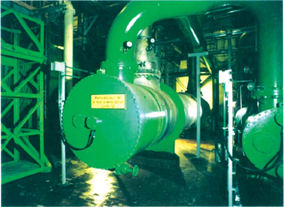
Fig. 9.5. Acid cooler, courtesy Chemetics www.chemetics.com Cool water flows through 1610 internal 2 cm diameter tubes while warm acid flows counter currently (and turbulently) between the tubes. The tubes are 316L stainless steel. They are resistant to water-side corrosion. They are electrochemically passivated against acid-side corrosion by continuously applying an electrical potential between the tubes and several electrically isolated metal rods. Details: shell diameter 1.65 m; shell material: 304L stainless steel; acid flow: 2000 m 3 /hour; water flow: 2900 m 3 /hour; acid temperature drop: 40 K. (Blue pipes = water; metallic pipes = acid.) Fig. 24.6 gives an internal view.
