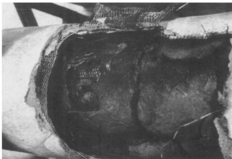
Figure 46. Results of fire test of a composite composed of U-modified isocyanurate foam and mortar (79). (Courtesy of Nisshin Spinning Co. Ltd.)
