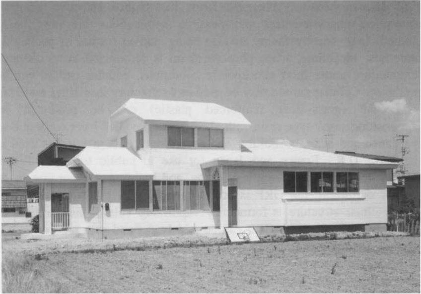
Figure 68. Wooden house employing metal-siding board as exterior material (Courtesy of IG-Industries, Japan).
