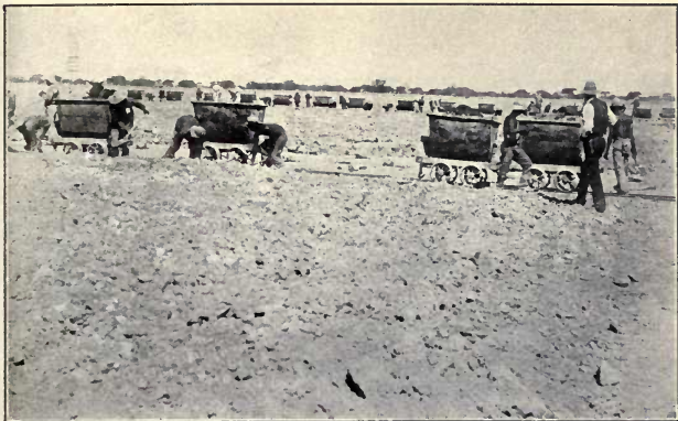
ON THE FLOORS LOADING BLUE EARTH FOR THE WASHING MACHINES, KIMBERLEY MINES
