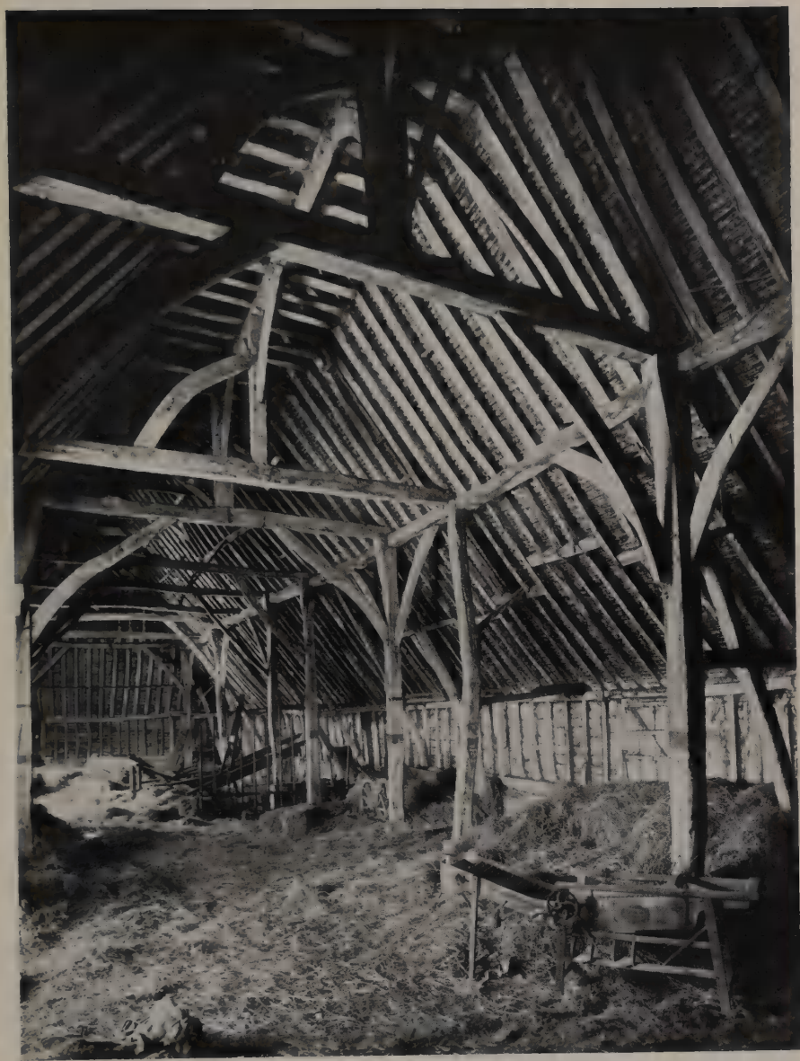
I. A MEDIEVAL TIMBER-FRAMED BUILDING The Barn, Court Lodge Farm, Godmersham
