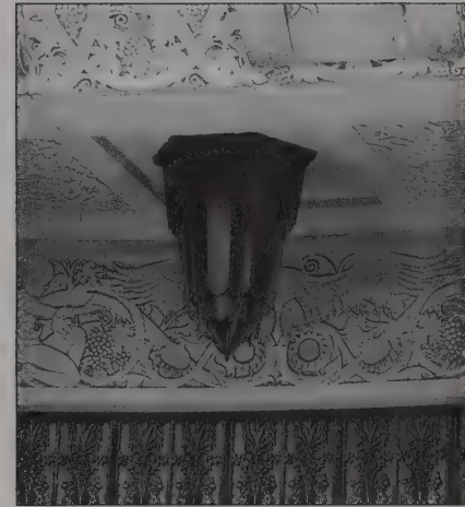
Mackenzie, Voorhees & Gmelin (architects): entrance detail, Barclay-Vesey building, corner of Barclay, Vesey, Washington and West Streets, New York, 1923-26. Considered ultra-modern by contemporary critics, the decoration on the terracotta frieze shown here looks distinctly Victorian in comparison to the angular ceiling fixture, which today appears far more advanced in concept.
