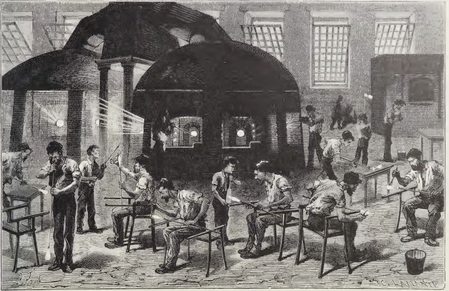
Interior view of a glassworks. (19th century engraving)
