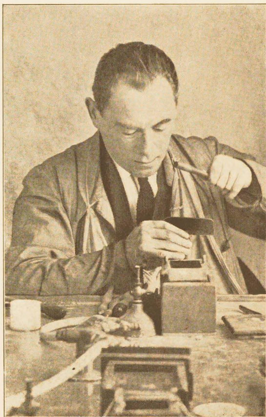
The cleaving of a diamond fixed in shellac.
