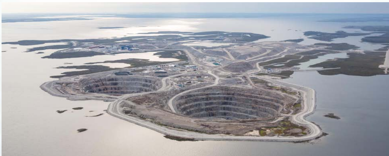
Figure 1: The Diavik diamond mine in Canada was initially underwater. A dyke allowed open pit working and currently it is being mined underground.
