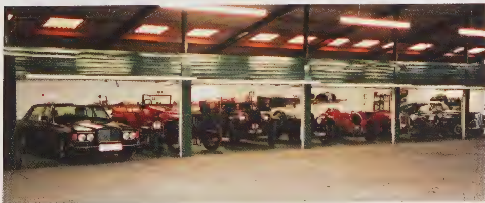
The completed lock-up garages within the huge barn.
