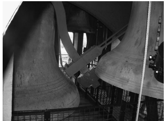
FIG 2.32 The hammer head is seen well away from the bell.
