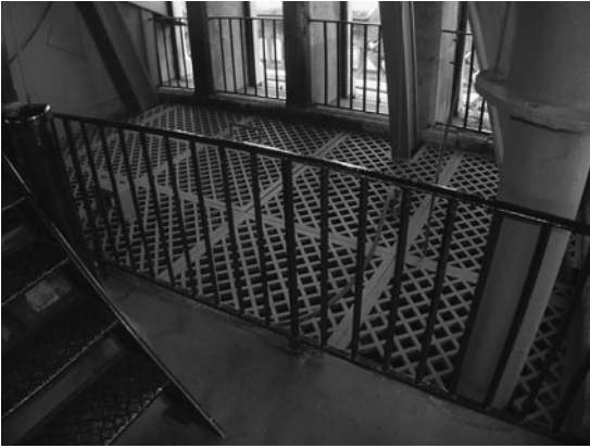
FIG 2.33 The top of the air shaft.
