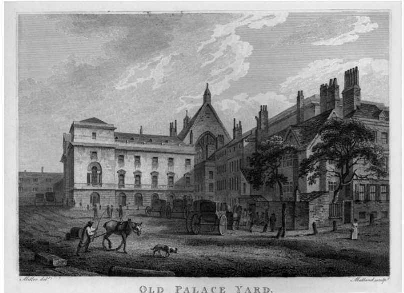
FIG 4.2 Old Palace Yard, 1796. In the background is the south end of Westminster Hall. To the right is the entrance to the House of Lords where the fire began. Del. Miller. Published Colnaghi & Co., 132, Pall Mall.
