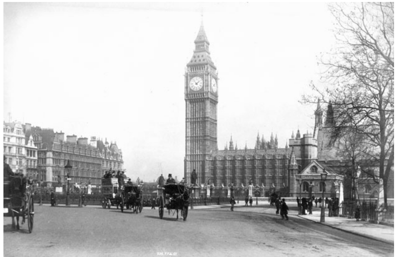
FIG 5.20 An albumen print of the Clock Tower, taken circa 1880, from Parliament Square looking across New Palace Yard. The stonework is in a clean condition, an indication that much of the pollution took place in the twentieth century.
