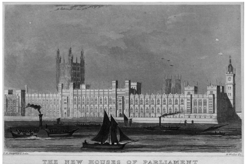
FIG 5.1 Barry's winning plan for the New Houses of Parliament. The Clock Tower was not a requirement of the competition but Barry added one after he was declared the winner.
