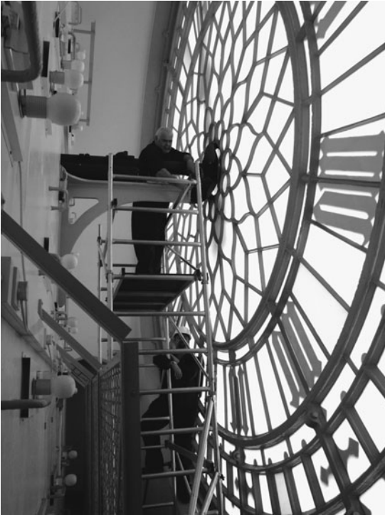
FIG 16.7 Scaffold behind dial to access the hour tube and minute arbor rollers.
