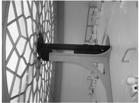
FIG 17.28 The cast-iron outrigger that supports the weight of the hands.
