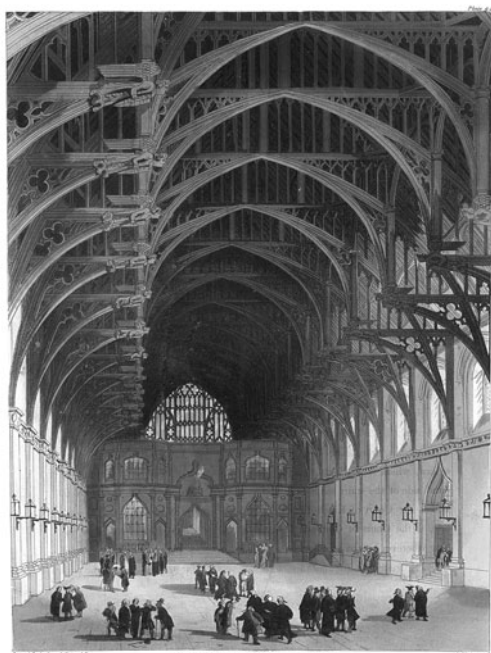
FIG 3.3 The inside of Westminster Hall, showing the magnificent hammer-beam roof. Etching and aquatint by Rowlandson and Pugin produced for the ‘Microcosm of London’ series, originally published 1808–10. This figure is reproduced in colour in the colour plate section.
