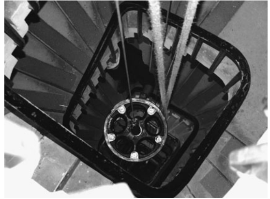
FIG 16.6 The striking barrel being lowered down the stairwell.
