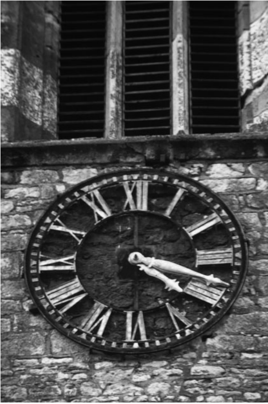
FIG 6.4 A skeleton dial of cast iron by James Harrison of Hull, North Cave church, 1851.
