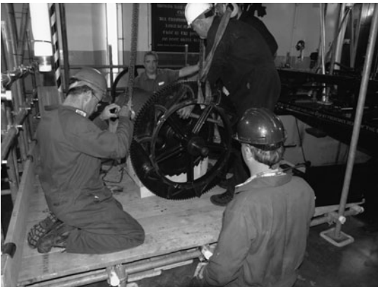
FIG 16.5 Safely in its cradle, the great wheel and arbor are removed from the hour-striking barrel.
