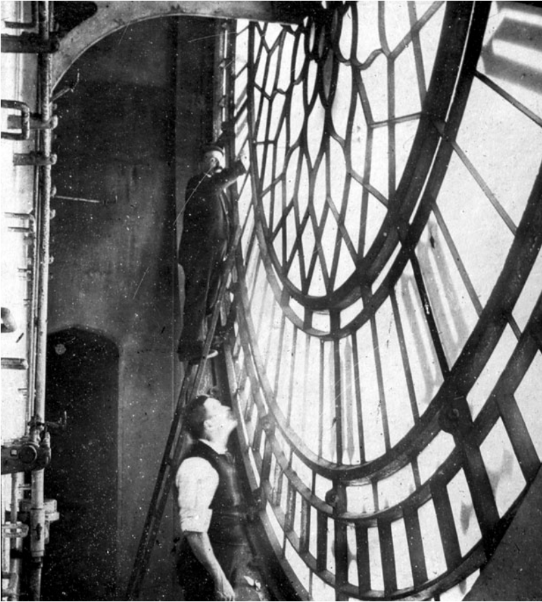
FIG 9.10 Cleaning the inside of a dial. A glass lantern slide shows two men working behind a dial. As there seem to be no electric lights fitted the picture, is pre-1905.
