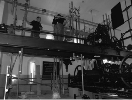
FIG 16.4 Erecting the scaffolding to enable the lifting of heavy parts.
