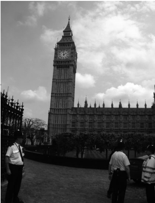
FIG 2.2 The Clock Tower from New Palace Yard. The entrance to the tower is through a passage between the tower and the main building.
