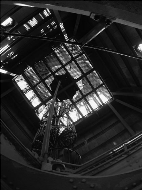
FIG 2.35 Looking up inside the spire.
