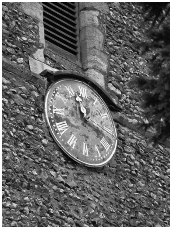
FIG 6.3 Painted copper dials were common from 1700 through to the 1960s, when glass-reinforced plastic replaced copper as a lighter and cheaper material.
