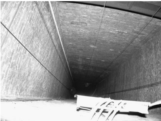
FIG 2.37 Weights can just be made out in the weight shaft below.
