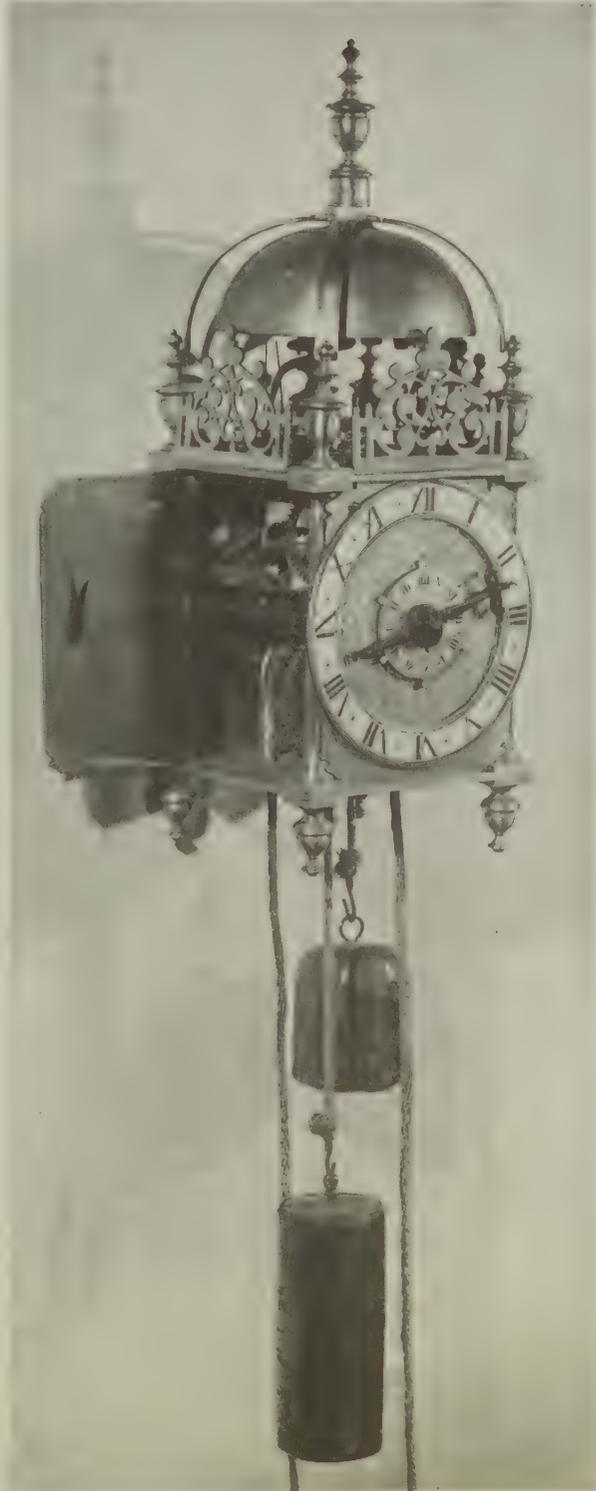
Two square bars can be seen in plate 9, about half-way up the side of the clock, extending from front to back and it is by arms at either end of these that the going train sets off the striking train at each hour.
