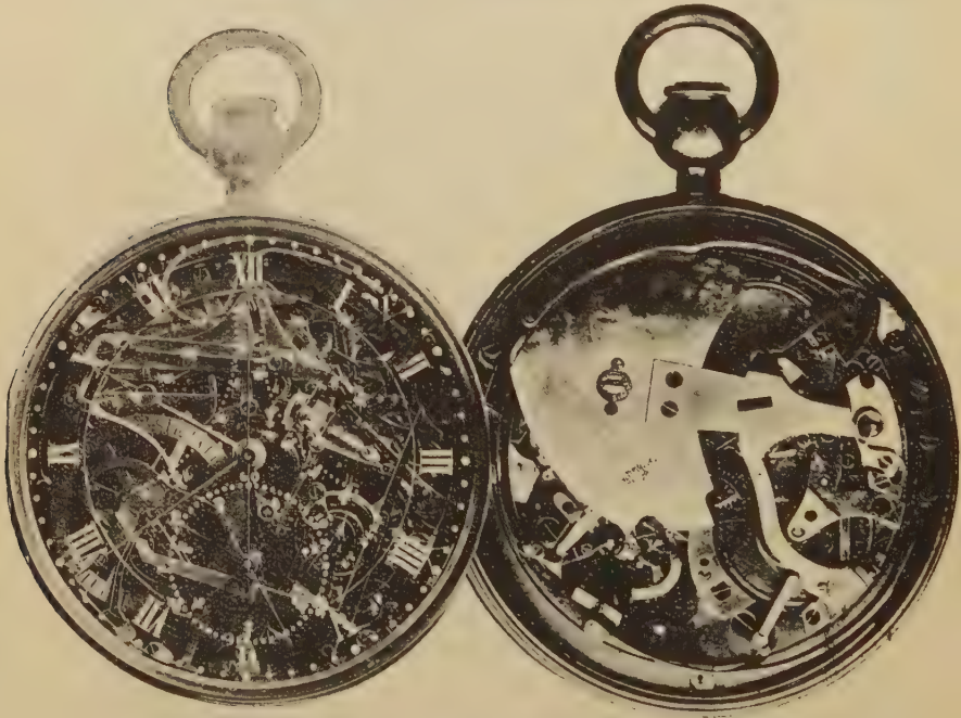
FIG. 565.—Breguet's " Chef-d'œuvre ," Perpetual or Self-Winding Watch with Gold Movement.
