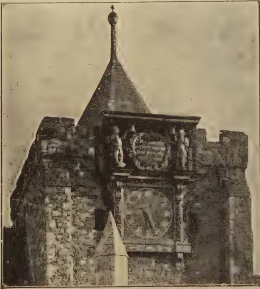
FIG. 21.—Jacks at Rye.
