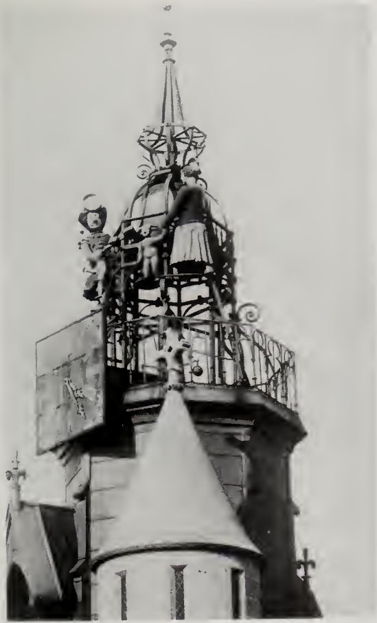
Human figures called jacks strike the hour and quarter-hour on this fourteenth-century clock in the Church of Notre Dame in Dijon, France.
