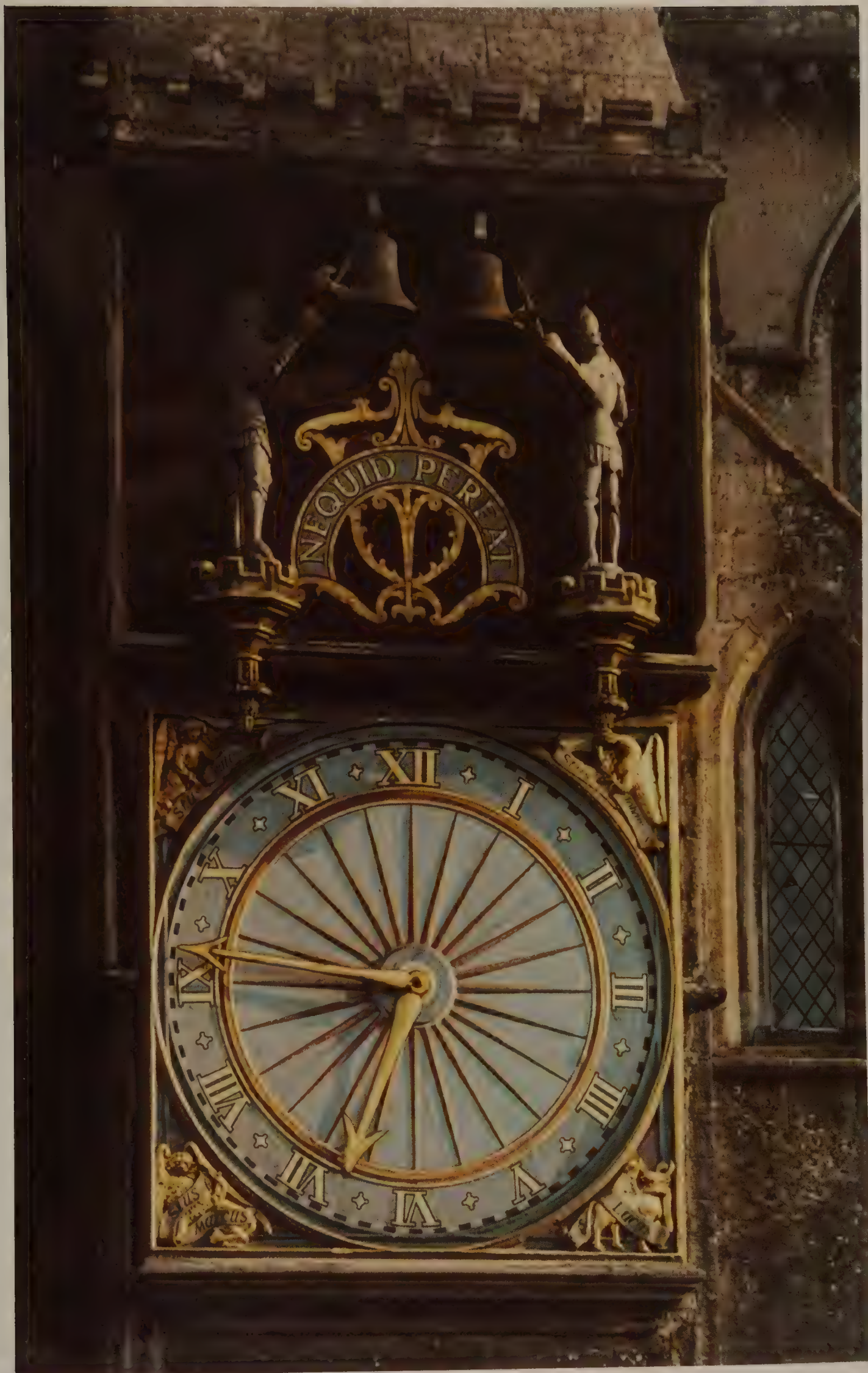
Right : The exterior dial of Wells Cathedral. The wooden jacks above it strike the quarters.
