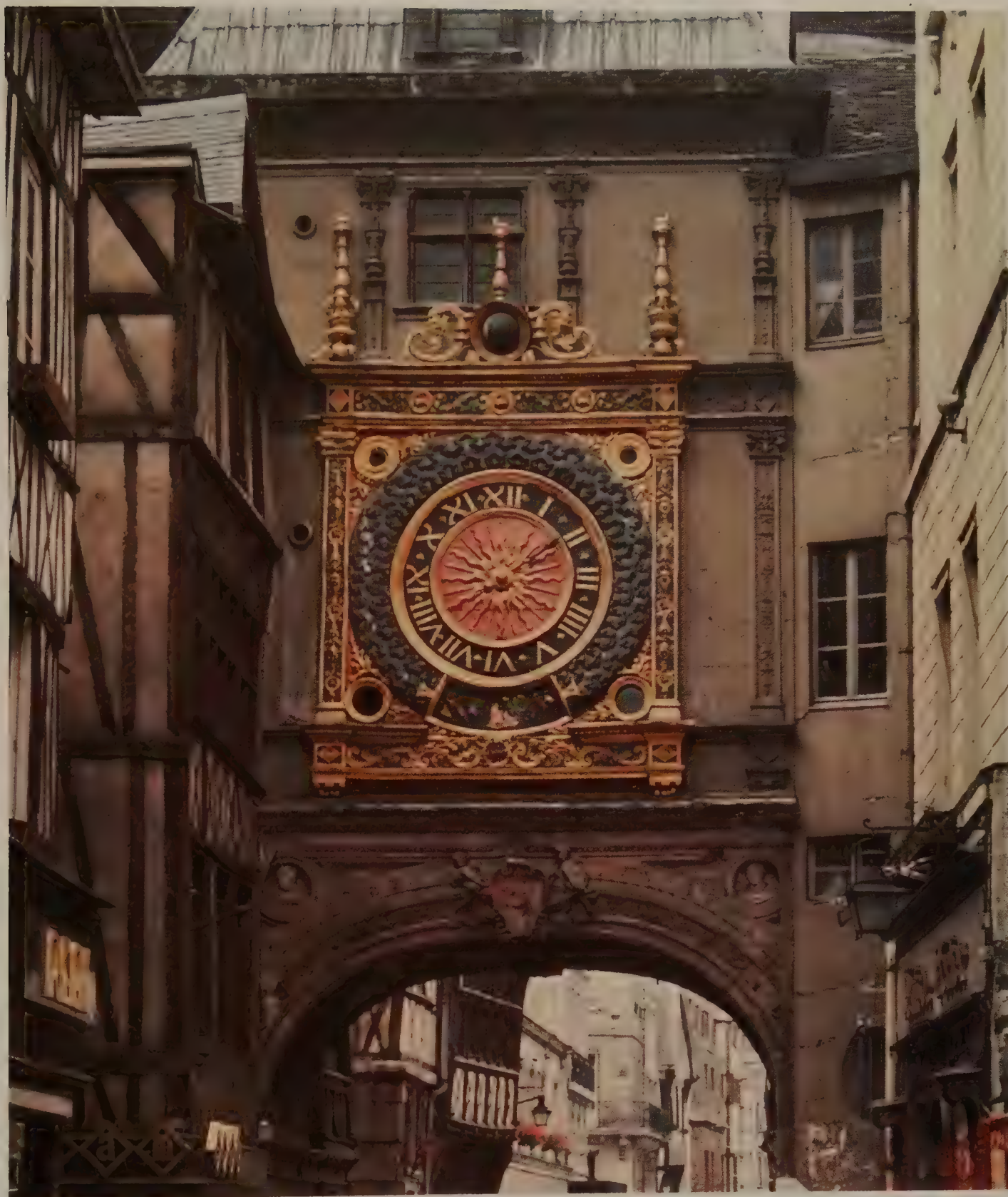
Right : The other Rouen clock dial (see page 234). At the top is a half black Moon which rotates to show the phase, and at the bottom the monthly signs of the zodiac. The carved wavy lines around the dial are a common symbol for clouds.
