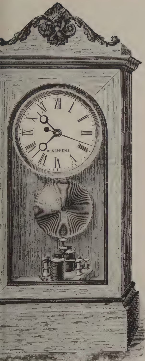
Above: Matthäu Hipp of Neuchâtel invented an ingenious toggle switch which much improved the performance of the electric clock because the pendulum was impulsed only when the arc fell off.
