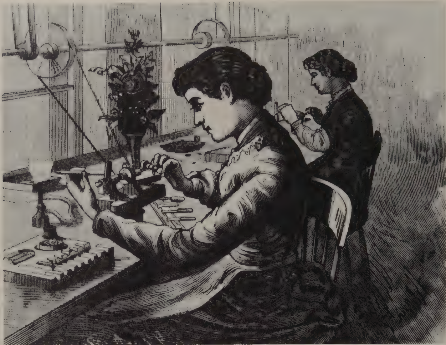
Right : Making jewel endstones and jewel holes out of ruby, sapphire and garnet at the Waltham Watch Works in 1885. Women, using gas flames to shellac the stones to the lathes, were employed because they could cope better, it was thought, with the fine tolerances involved.
