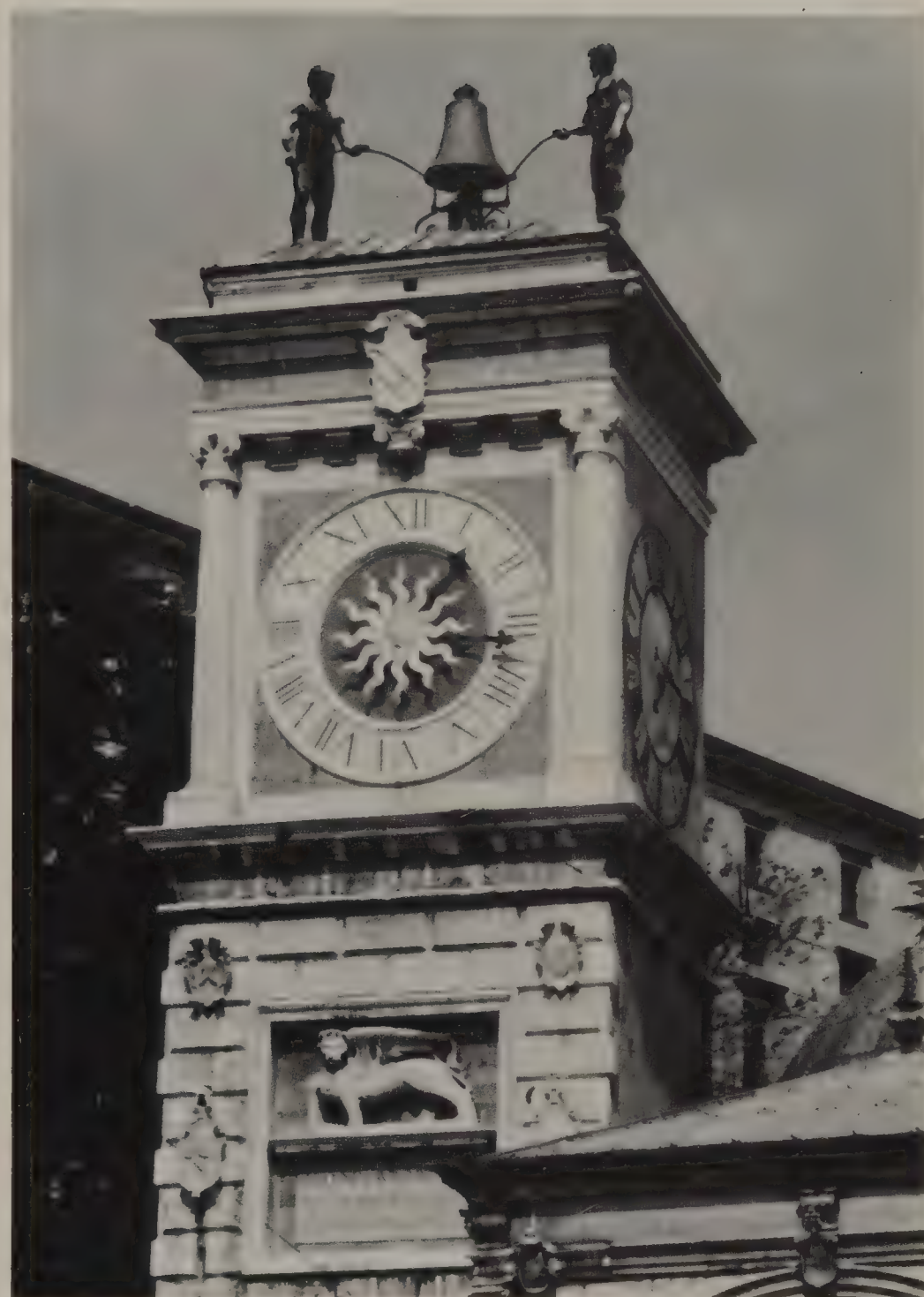
Above: The clock in the church tower (1527-30) in the Piazza della Libertà, Udine, Italy, which has two jacks striking a bell alternately. The original wooden jacks were made about 1393, the present copper ones in 1850.
