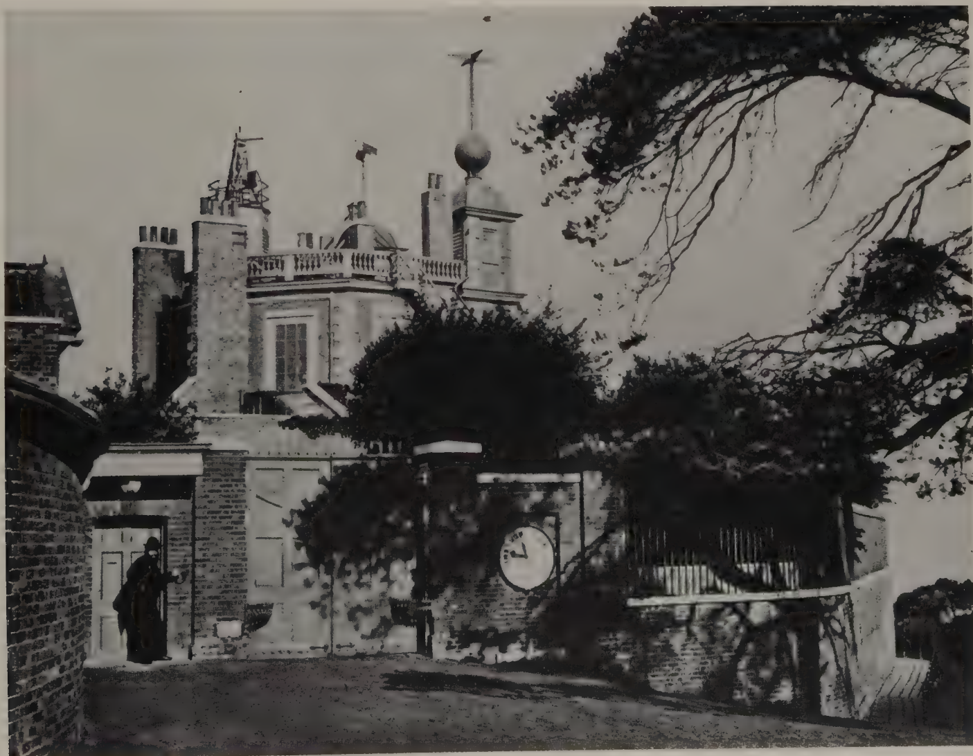
Right : Greenwich Observatory with Shepherd's clock, installed by Airey, and the time ball on the roof, which dropped at noon to signal time to shipping in the Greenwich Reach.
