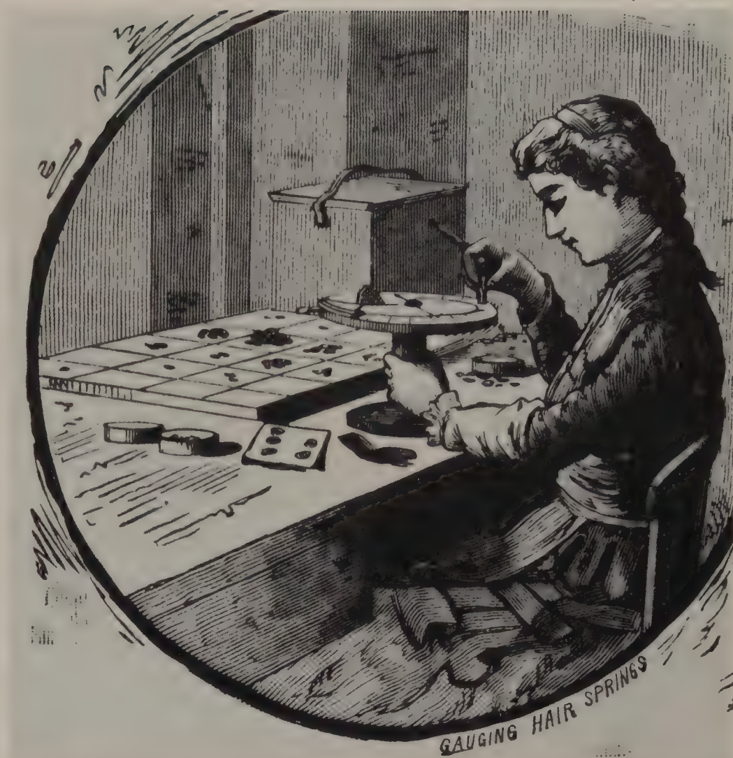
Above: Women also handled the delicate hairsprings, under large windows for daylight, and gaslights, or the rare incandescent electric lamps, by night.
