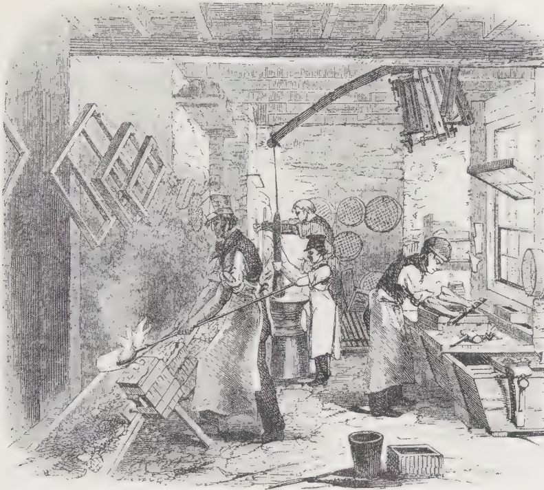
Plate 120 The J. Smith brass foundry where plates and other parts were cast.
