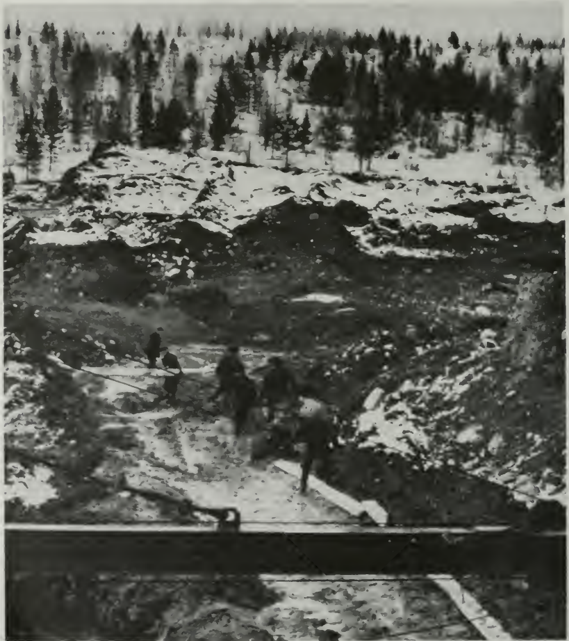
A view of a Siberian diamond mine showing workers digging in the frozen ground. (His Excellency Mr. Arnold Smith.)
