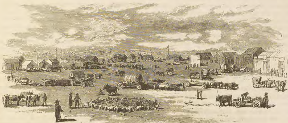
DU TOIT'S PAN—MARKET SQUARE.
