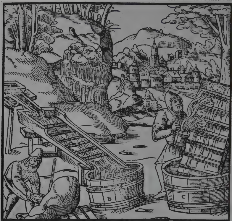
Fig. 4.2. The Long Tom, introduced to South Africa by Australian diggers, has a very long history. This picture shows it in use; it comes from Re de Metallica by Georgius Agricola, published in 1550.
