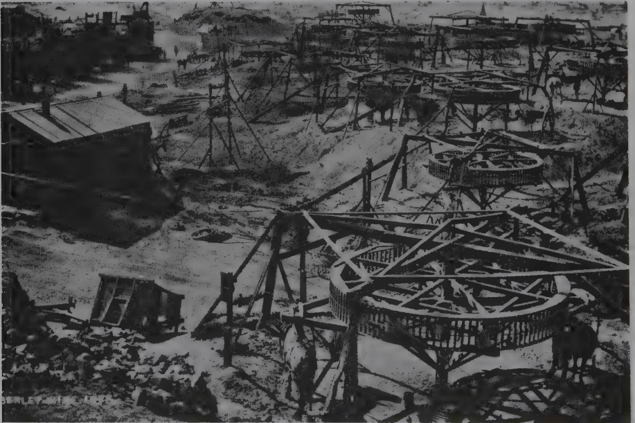
Fig. 4.17. The top edge of the Kimberley mine in 1878 showing whims turned by horses to draw up the buckets of ore.
