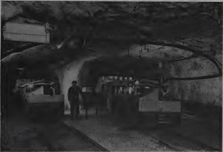
Fig. 4.33. Granby trucks used for taking blue ground to the underground crushing plant at the Premier Mine.
