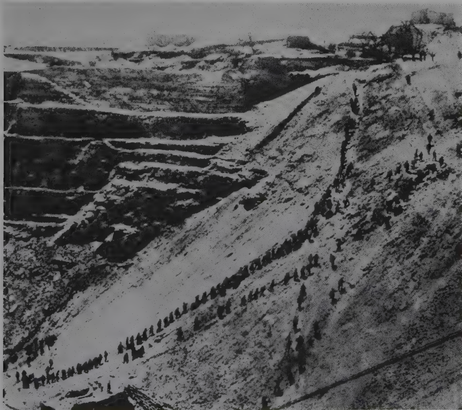
Fig. 4.9. Chains of labourers working in the west side of the De Beers mine when it was still worked by open cast methods.
