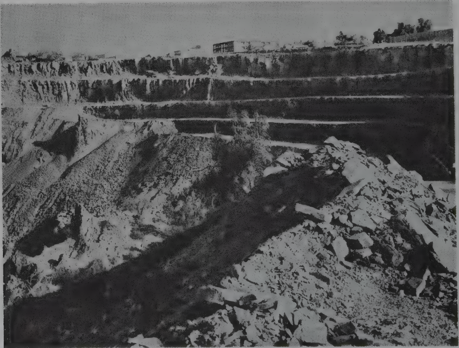
Fig. 4.24. A five-year operation, during the 1960s and 1970s, terraced the top of De Beers mine to stop overburden from falling in. About 25,000,000 tons of rock were moved.
