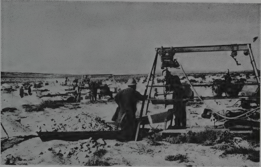
Fig. 4.43. Rows of prospecting holes, first made by the drill in Fig. 4.42 and lined with steel casings, which have been taken into the gravels and are being sampled using a small crane and a bucket. One man is working underground.
