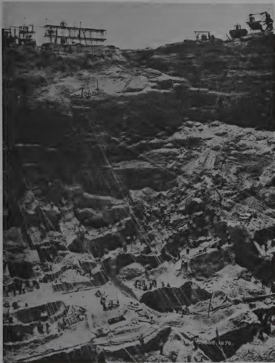
Fig. 4.15. Staging in several tiers round the edge of the Kimberley mine in 1878 to hold the cables up which hide and metal buckets of ore were drawn. It was like a giant cobweb.
