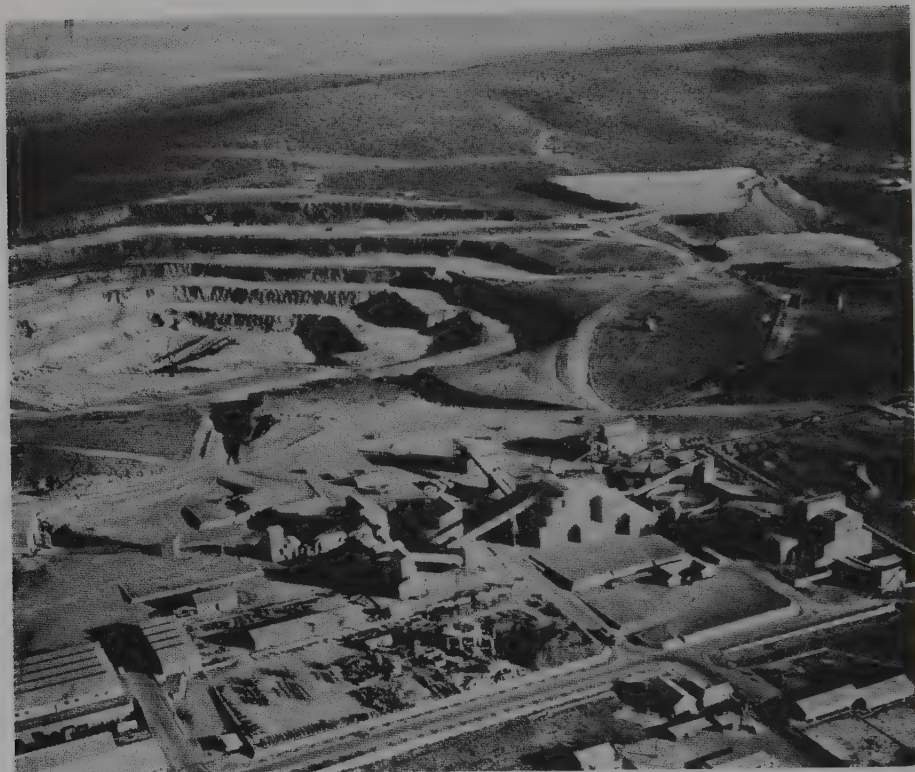
Fig. 4.34. The Finsch pipe from the air. It is being worked by open cast methods. The treatment plant is in the foreground. The pipe is at Lime Acres.
