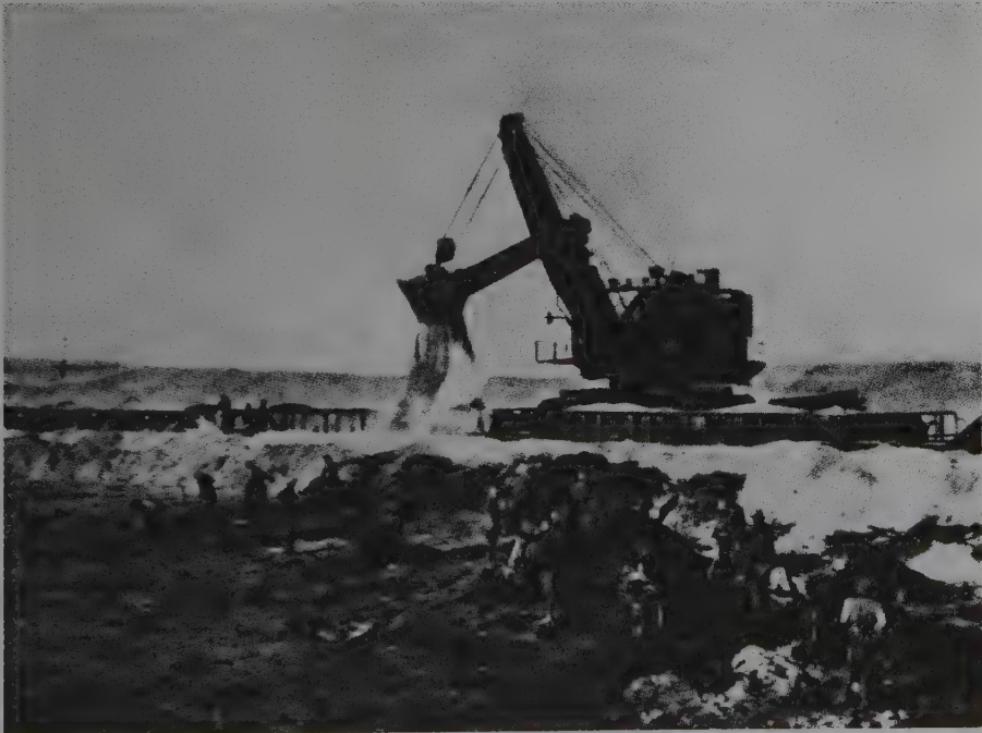
Fig. 3.23. After Consolidated Diamond Mines took over they introduced more mechanical means of stripping the sand from beaches. This was at Elizabeth Bay.
