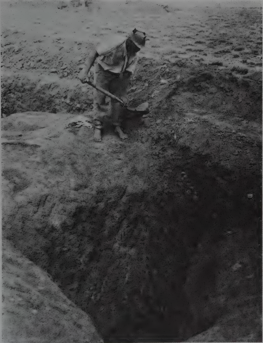
Fig. 4.1. Digging a prospecting pit at the corner of a claim to determine the depth of the layer of diamondiferous gravel.
