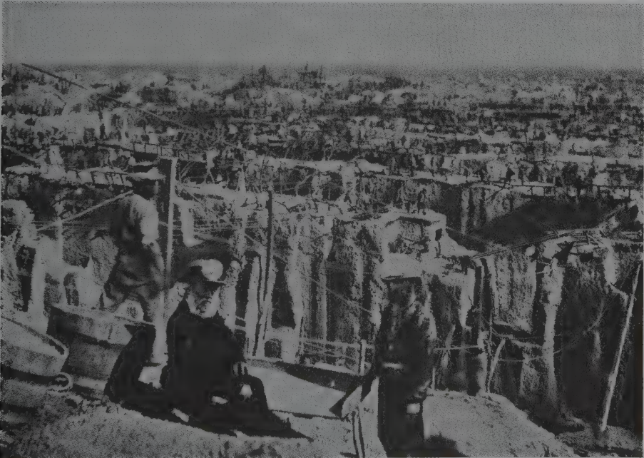
Fig. 4.12 Another view of Kimberley when the 'roads' were beginning to collapse. The buckets in the foreground were lowered to be filled with ground. In the background can be seen dumps on the edge of the Big Hole and staging being built.
