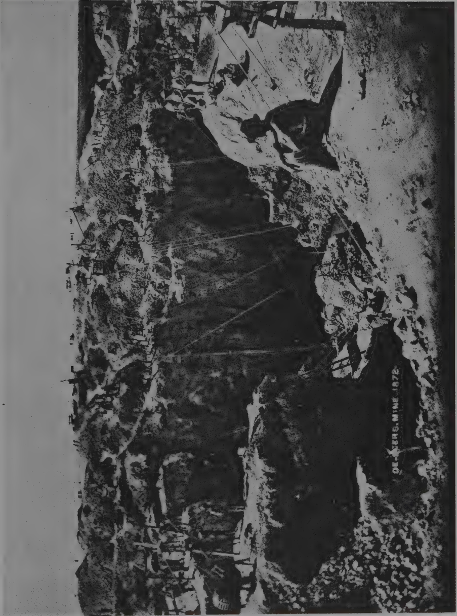
Fig. 3.9. De Beers mine in 1872, after it had become so deep that cables and buckets had to be used to bring up the ground. A man winding up a bucket can be seen on the left.
