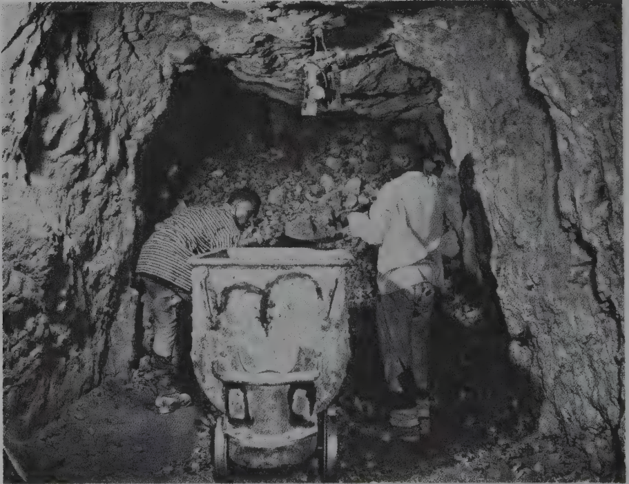
Fig. 4.29. Loading blue ground into a hand truck after chambering.
