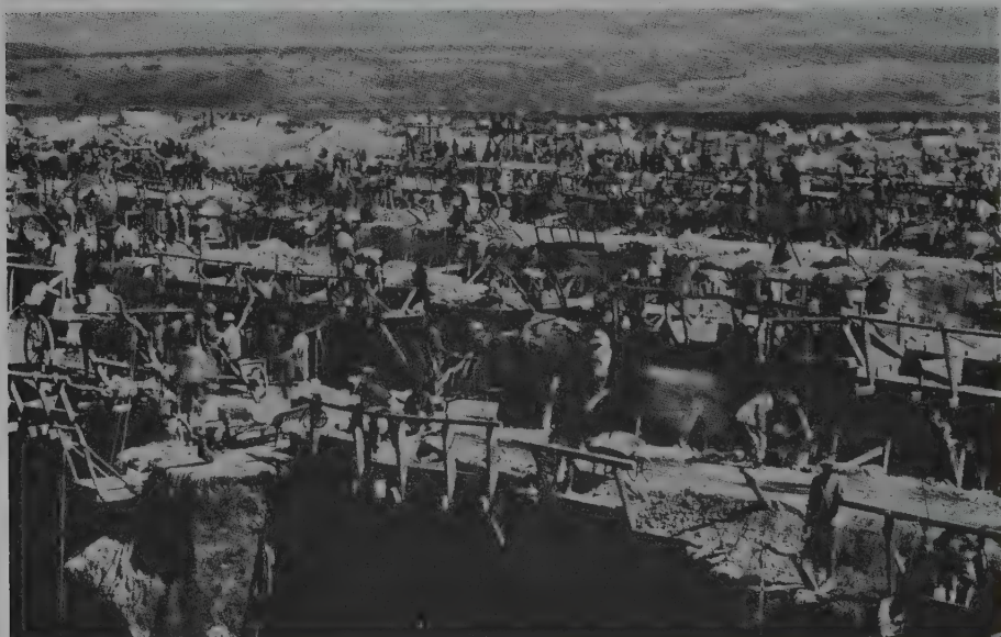
Fig. 4.11. The Kimberley mine in 1872 when roads left between claims were beginning to crumble at the edges.
