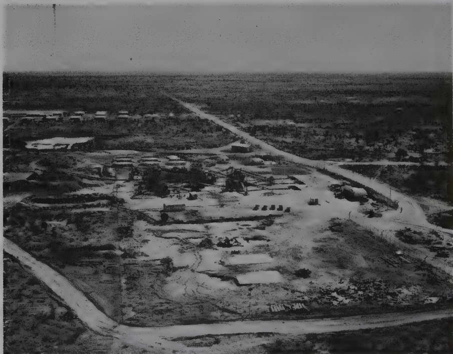
Fig. 6.8. The pilot treatment plant set up at the Orapa diamond pipe in central Botswana to treat about 275 tons a day. The pipe, developed by De Beers, came into full operation in 1971 and now produces about 2,500,000 carats a year.
