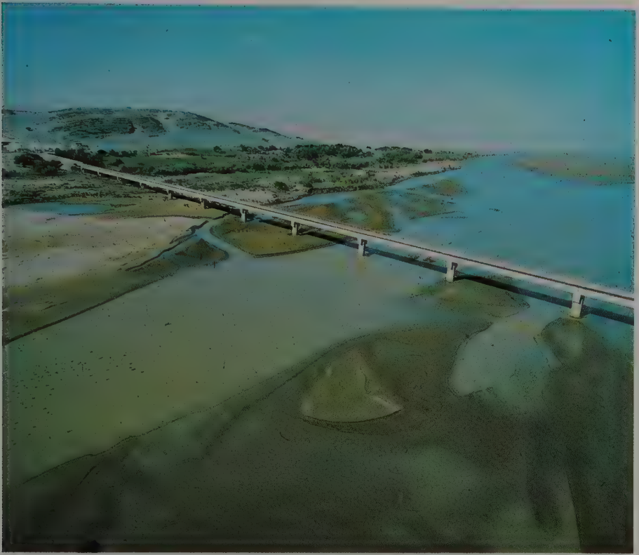
The Ernest Oppenheimer Bridge over the Orange River, that connects South Africa with the diamond-bearing coastal desert of Namibia (South West Africa).
