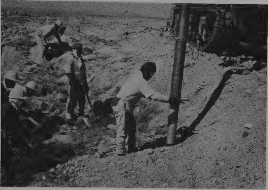
Fig. 4.40. A suction hose called the Vacuveyor or bedrock cleaner was used at one time to empty potholes of sand and gravel.
