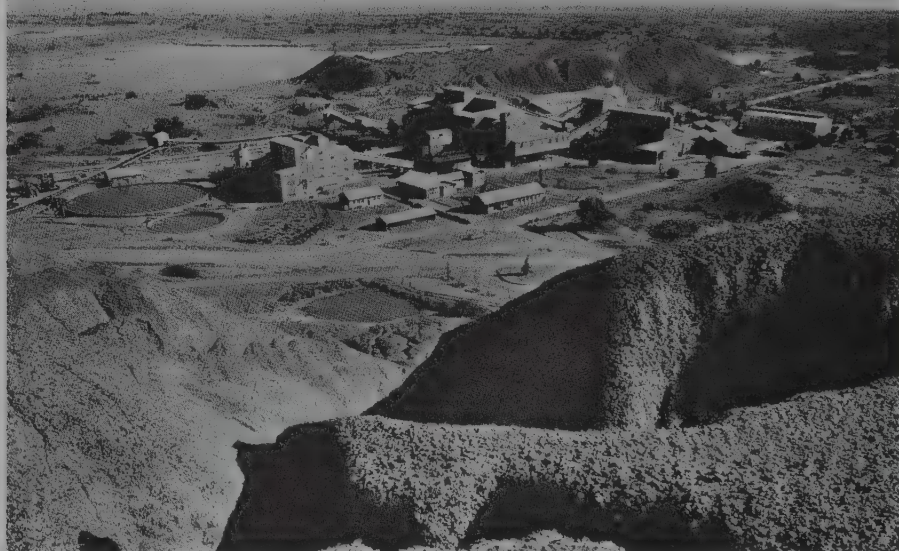
Fig. 5.3. The central treatment plant at Kimberley which extracts diamonds from the pipe mines. The waste material - the tailings - is dumped near the plant as seen in the foreground.
