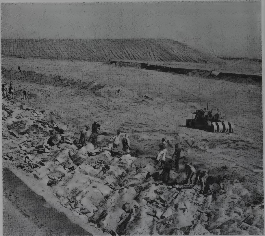
Fig. 4.38. The sand has been removed in the middle distance and piled in the far distance. The scraper has piled up diamond-bearing gravels on the left (upper left to centre of picture). In the foreground, the bedrock is being cleaned to remove any remaining gravel.
