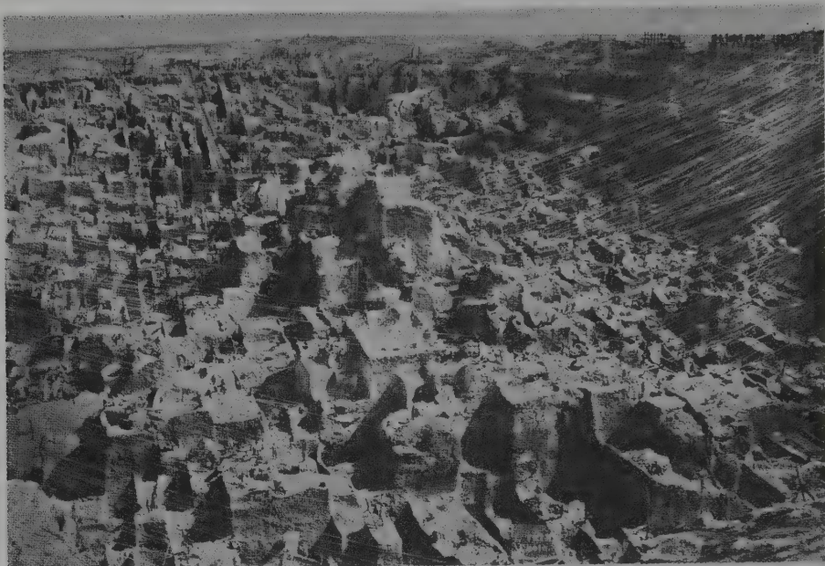
Fig. 4.13. The Big Hole in 1877. Note the ladder leaning on the centre block and the staging on the right. Near the top, about quarter of the way across the picture from the left, is the runway of a trolley system, perhaps the one in Fig. 4.19.
