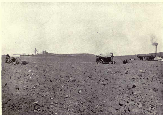
LOADING THE BLUE GROUND ON THE FLOORS, AND PLOUGHING IT OVER
