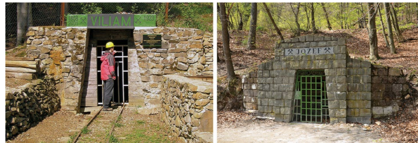
Figure 12. Left: Entrance portal to the Viliam hereditary adit (2011). Right: Entrance portal to the Jozef adit (2014). Photos the Author.
