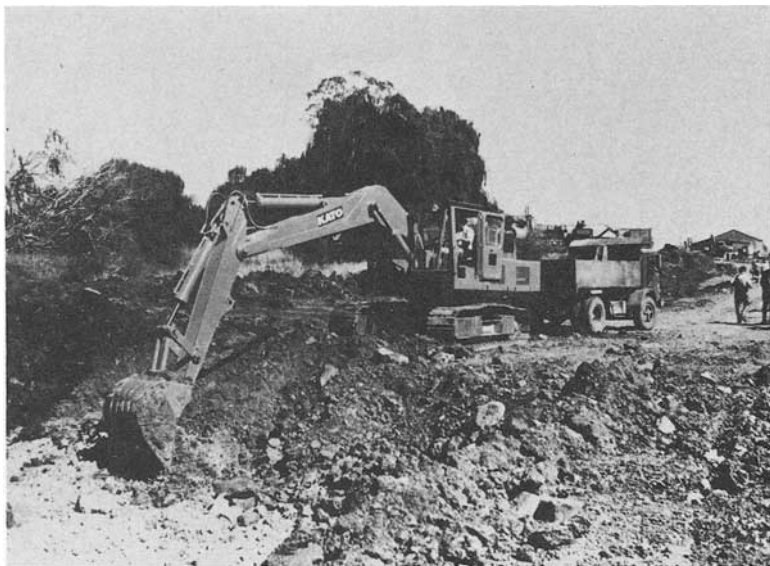
FIG. 3. Excavation of the sapphire-bearing gravels at the Stellar mine on the Horse Gully.
