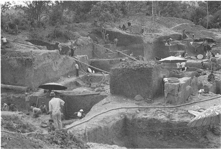
FIG. 4. Open cut workings in alluvium near Pailin. Note the stepped rectangular pattern of excavation, the competent vertical faces of the alluvium and the dumped overburden in the background.
