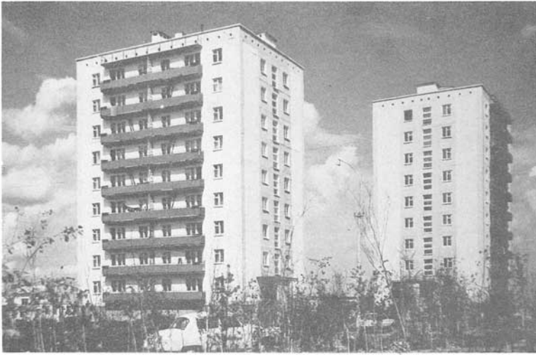
FIG. 5. Workers' flats at Mirny (summer): about 1980.
