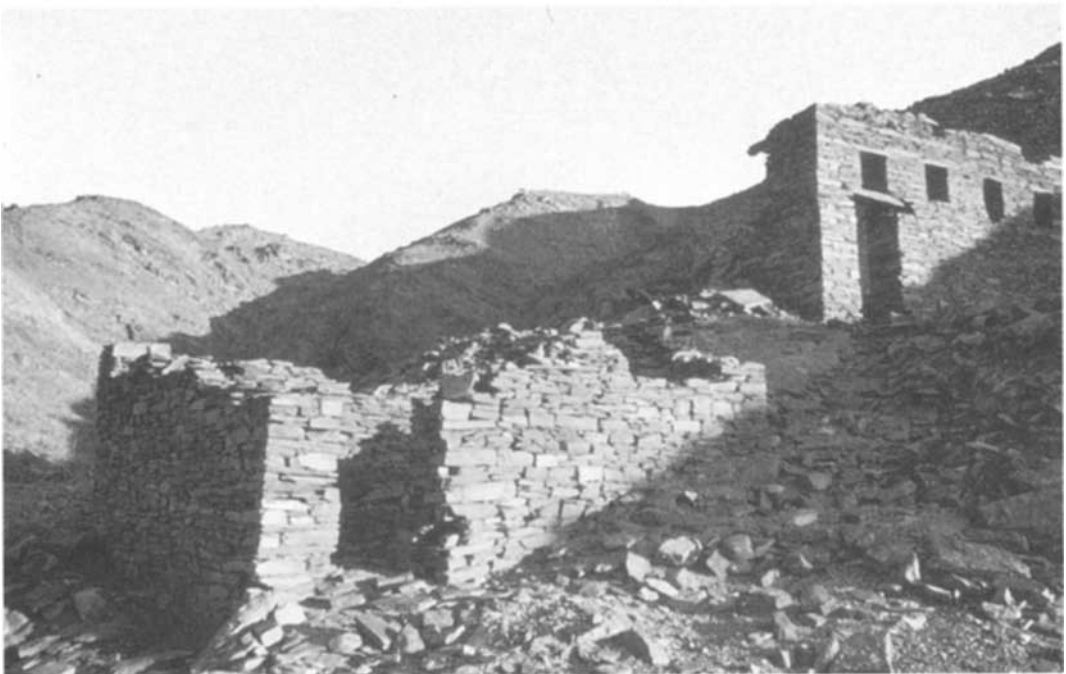
Fig. 3. The ancient residences of Sikeit miners. The ruins of the houses are scattered on two sides of the mountains which flank the valley. The constructions show a great accuracy of execution: the stones, without mortar, are accurately selected in order to fit in one another to form a compact, smooth and exactly vertical wall.
