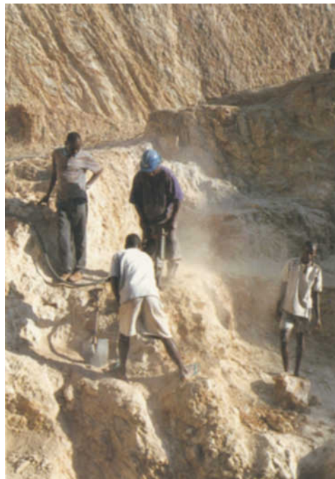
Figure 4: Working on the pegmatite vein at the Yellow Mine using jack hammers; no explosives are used.
