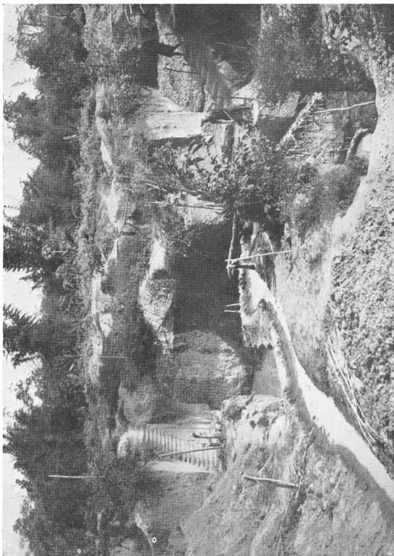
Fig. 2. — Typical zircon mine. Right — digging. Centre — washing earth away.
