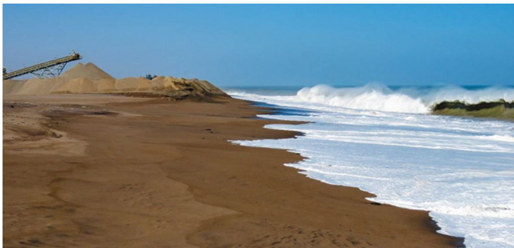
Figure 8: In order to increase the land surface, beach accretion takes place by moving sand from the interior onto the beach. Wave action aids in transporting the sand along the beach. Photo by J. Jacob.
