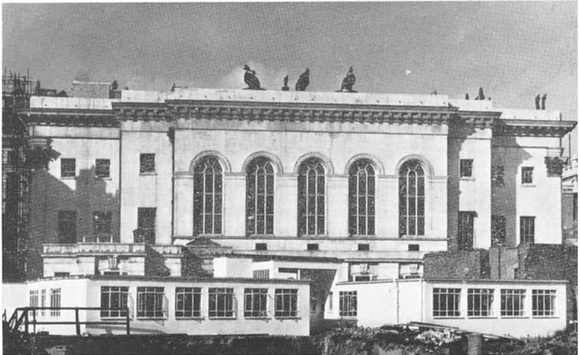
The temporary building which houses the Headquarters of the National Association of Goldsmiths, British Jewellers' Association, the National Jewellers' Association and the Gemmological Association of Great Britain. Behind is the facade of Goldsmiths' Hall.
