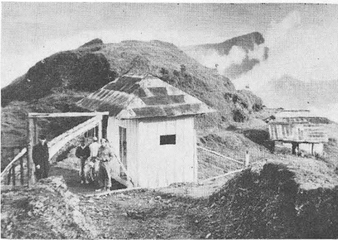
FIG. 3. Main entrance to the Chivor Mine, which is guarded at all times by the Colombian National Police. The wooden flume framed by the mine gate is part of the canal which brings the water from a river source 18 kilometres from the mine.
